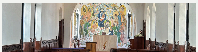
The Chapel now under refurbishment and roof repair
